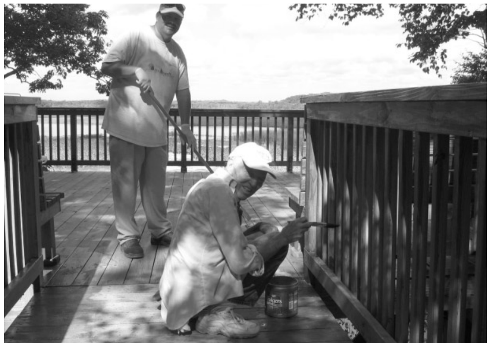
Maintenance staff John Evans and Frank Speaks put a new coat of stain on the Observation Deck.
